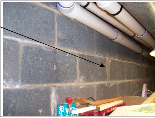
Horizontal Cracking Rear Foundation Wall of Garage
