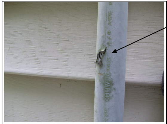
Main Cable Damaged
