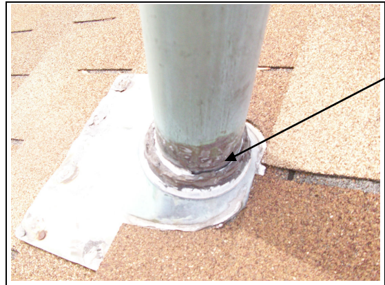
Gap at Vent Pipe Flashing
