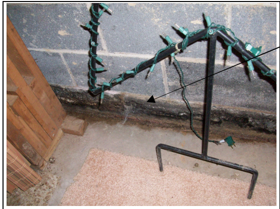
Possible Mold in Basement on Walls
