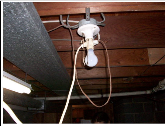
Extension Cord Wiring in Basement
