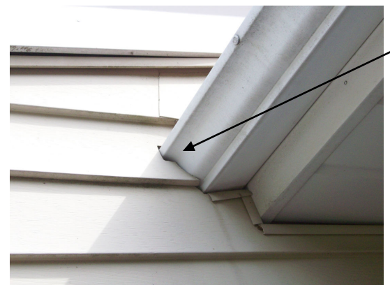
Gap at Siding at Gutter Rear of House
