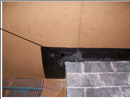
Prior Water Damage in Garage at Chimney
