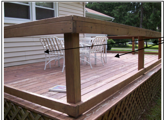
Deck Railing Low & Openings Too Wide
