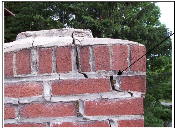
Damaged Mortar Joints && Loose Bricks
