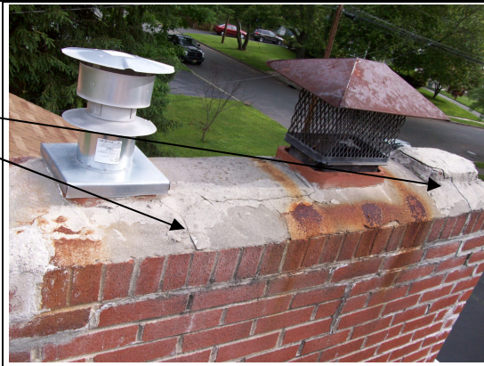
Cracked & Damaged Chimney Wash
