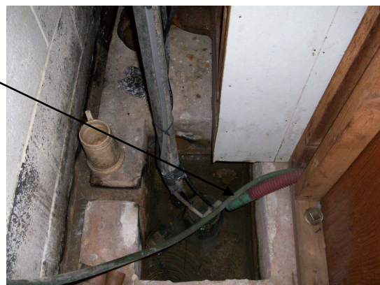
Bar Drain in Sump Pit
