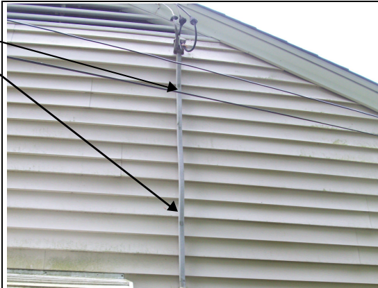
Clamps Needed on Main Cable
